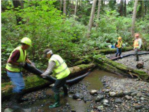
1.) QBSS crew setting up sediment control
