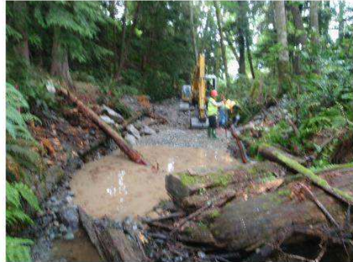
3.) Construction process August 2013
